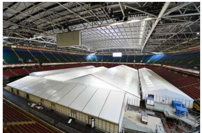
Dragon Heart Hospital time-lapse video of construction
